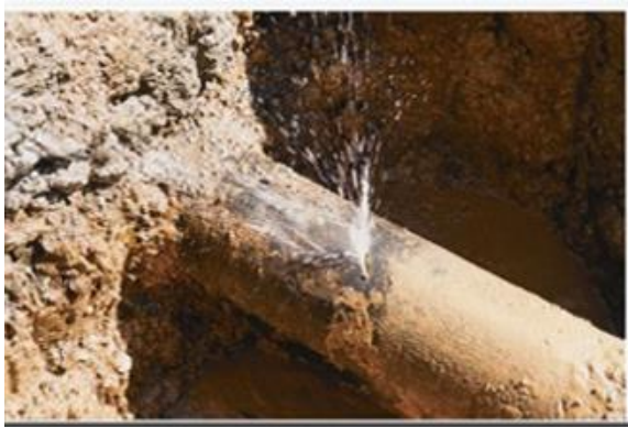
Figure 1. Metal pipe water leakage
