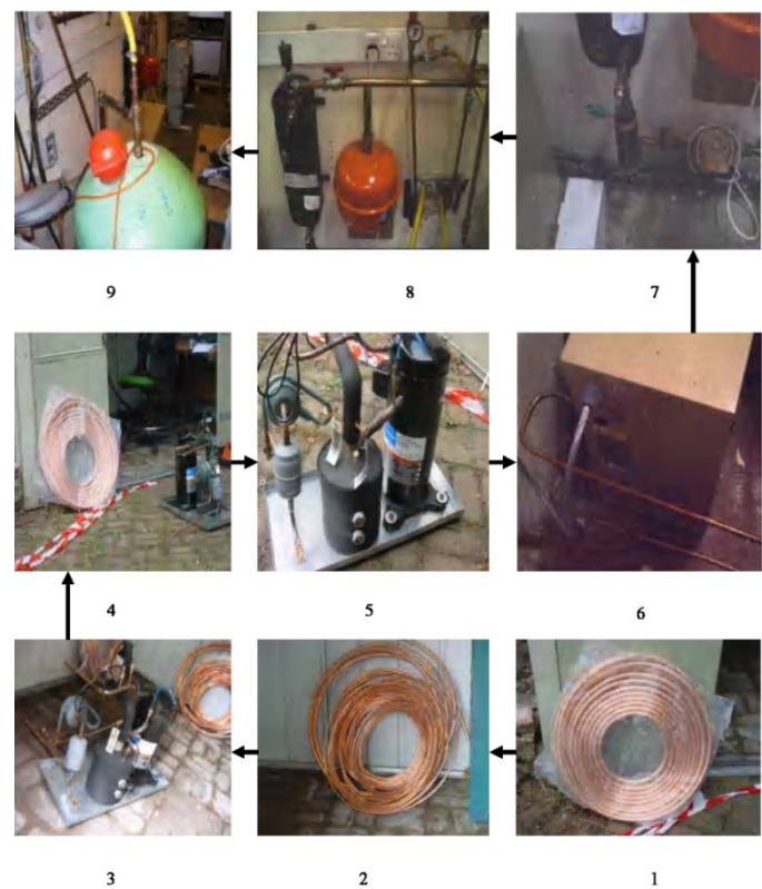
Figure 4. Showing preparation of coils (1-2), installation of heat pump (3-6) and connection of water supply system (water pump, flow metre, expansion valve and the boiler) (7-9).
